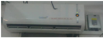
Coolsure UTS-36W Air Conditioner with BCU4818
